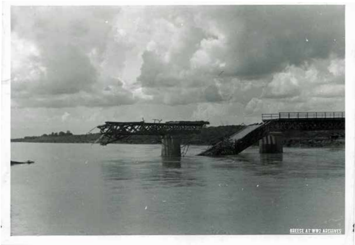
Fig. 8. Photograph of the Niseli road bridge over the Aliakmon river, following its destruction by New Zealand engineers in April 1941 (photograph 165982568_3577659632343862_1922733958124551261_n.jpg from "Greece in WW2 Archives", accessible at https://www.facebook.com/GreeceAtWw2Photostory/posts/pfbid0361obHffW2LxbmngqoGFGCJMLDxpMEqiQJa7YecV55ehCuMEuFvjzjn6zmsZV8gBl ).
